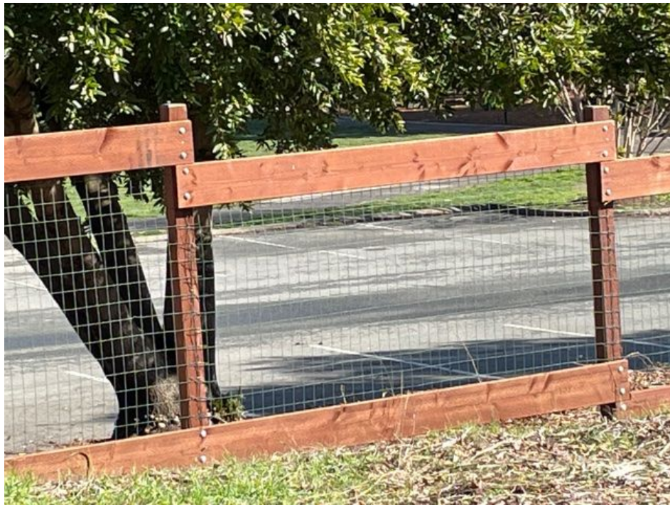
Remesh wire and redwood fencing allows for maximum visibility and in keeping with rustic setting.
